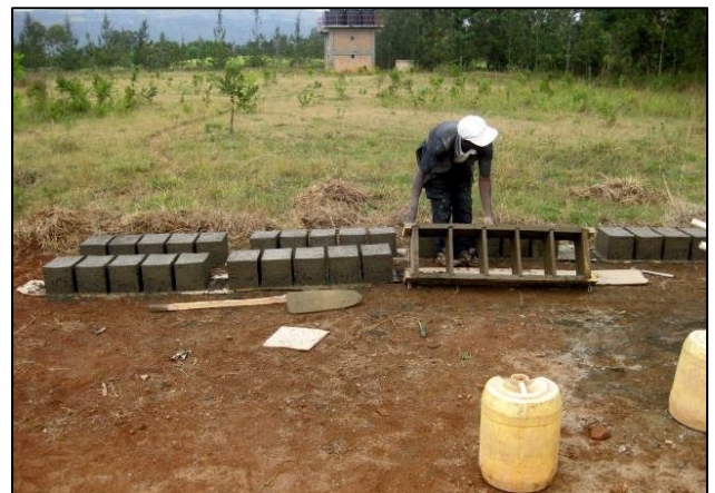
Making cement blocks (200 per day)
