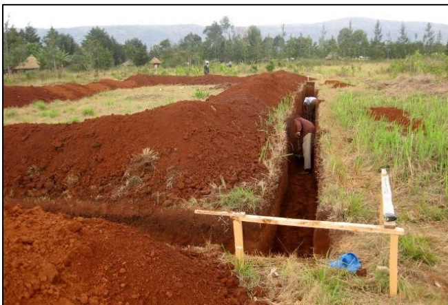
Trenching for Multi-purpose hall
