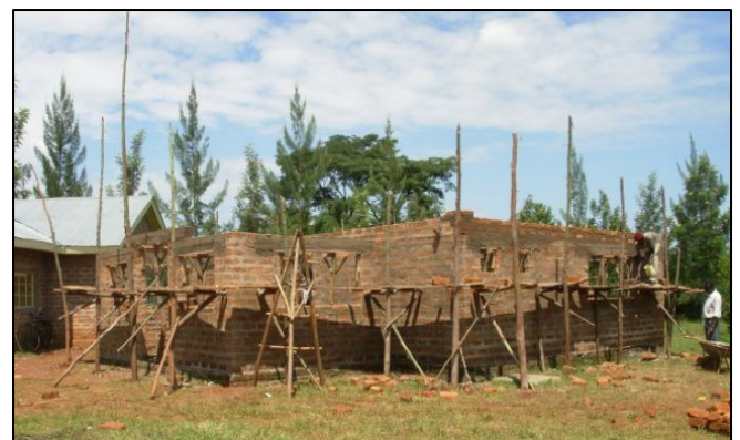
Construction started on 2 nd house in Malava
