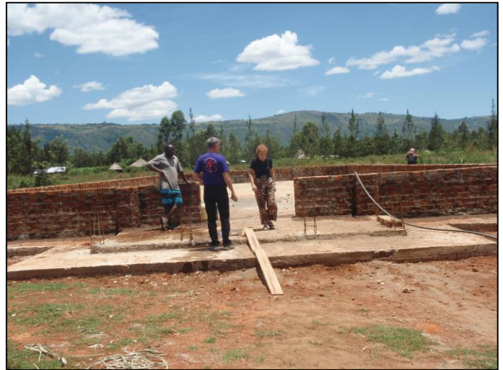
The walls are going up!
